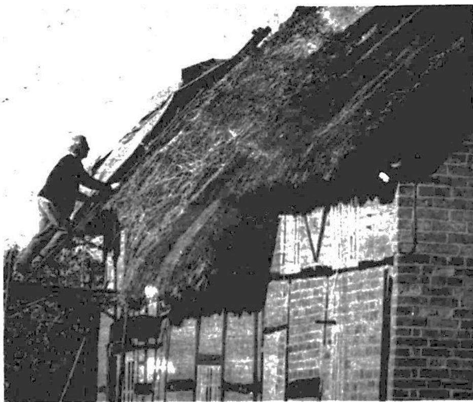
Work starts on repairing the thatched roof of the old cottage at Stoneleigh village, near Coventry. The cottage was recently damaged by fire.
