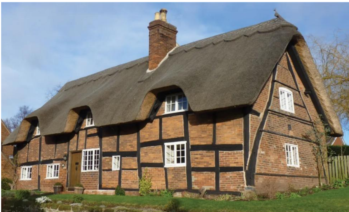
Phoenix Cottage in Stoneleigh Village - showing Cruck Construction
