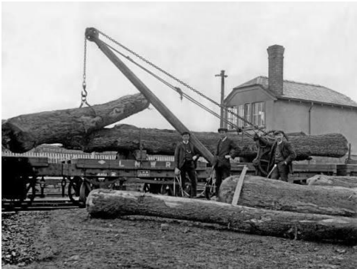
London North Western Railway - Pole Wagons
