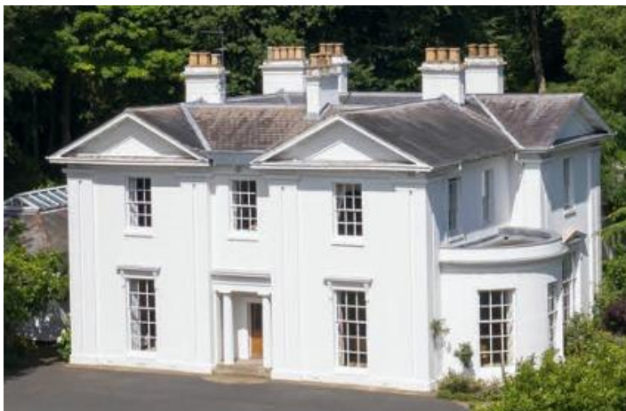
The Birches, Hagley, Stourbridge. A Grade II listed Georgian home set within 19.64 acres.
