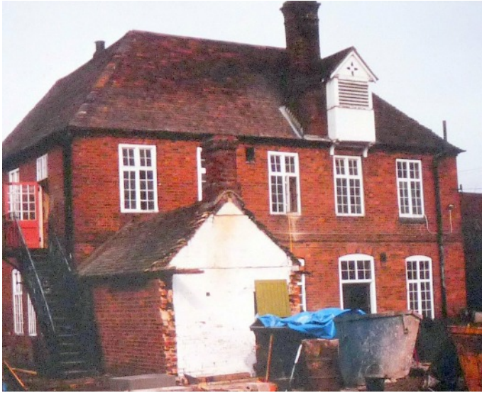
The school under demolition. Picture courtesy of Shirley Ball.
